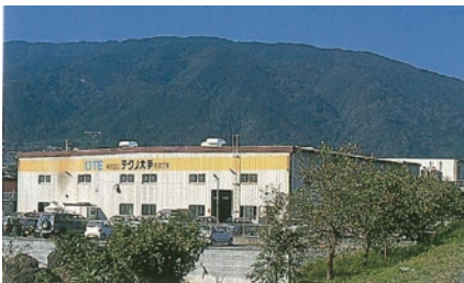
OTE Technological Engineering Corporation, Gifu Plant
